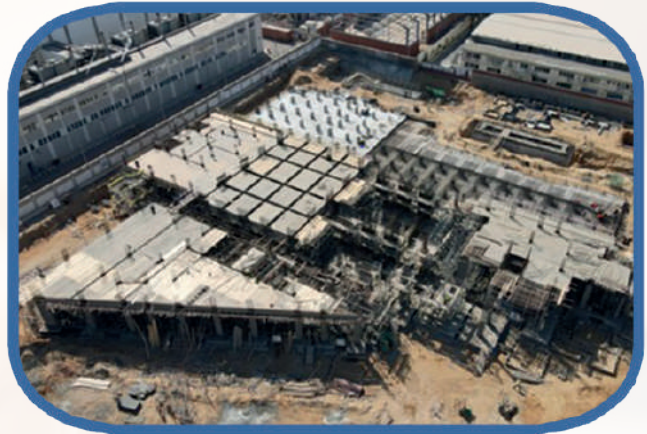
Progress Photo for the site in 2022
